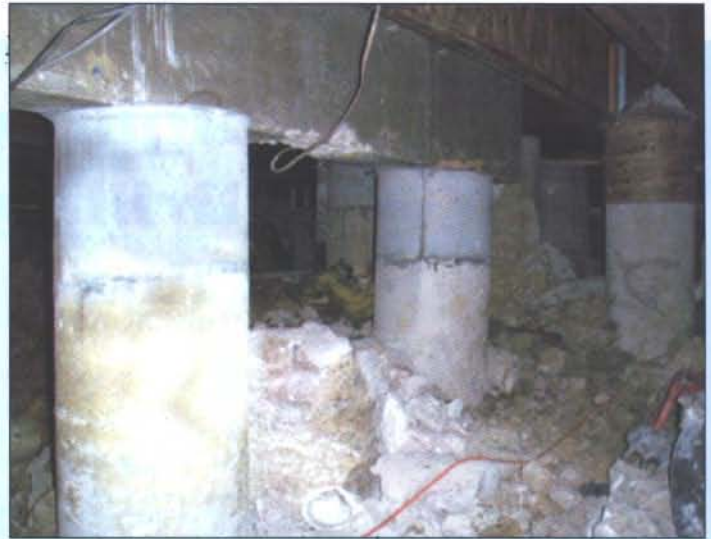
Finished pier columns up under foundation.
