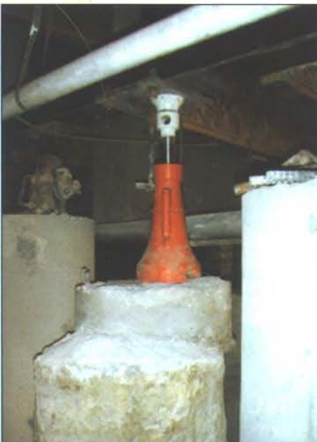
Screw jack set in place.
