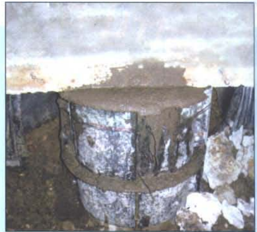
Pier cap poured under beam.
