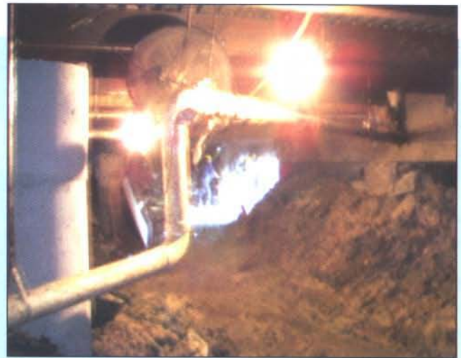
Main access route.
