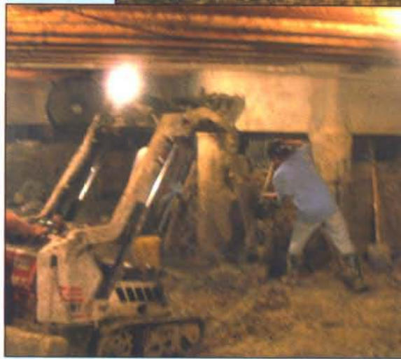
Drilling under concrete beams.
