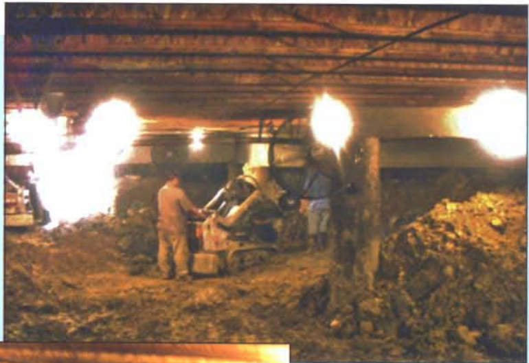
Excavating under the building.
