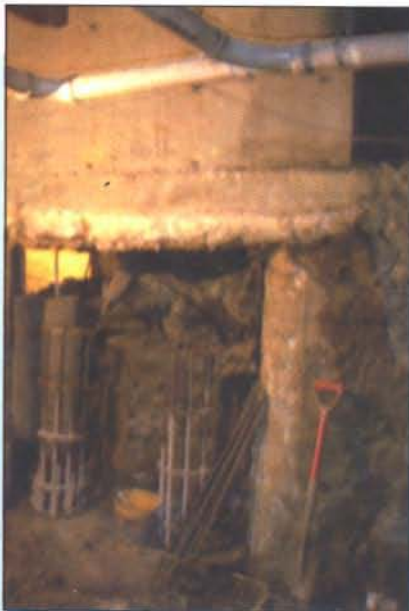
Steel extended up from piers.
